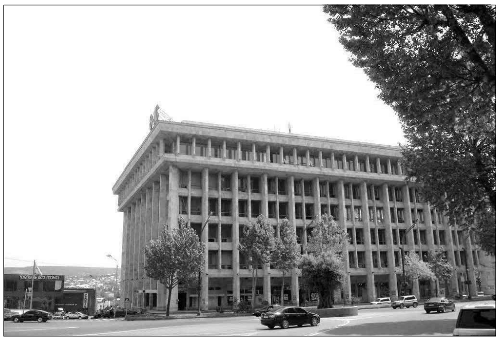
Radisson Blu Telegraph Hotel RUSTAVELI AVENUE, TBLISI, GEORGIA
